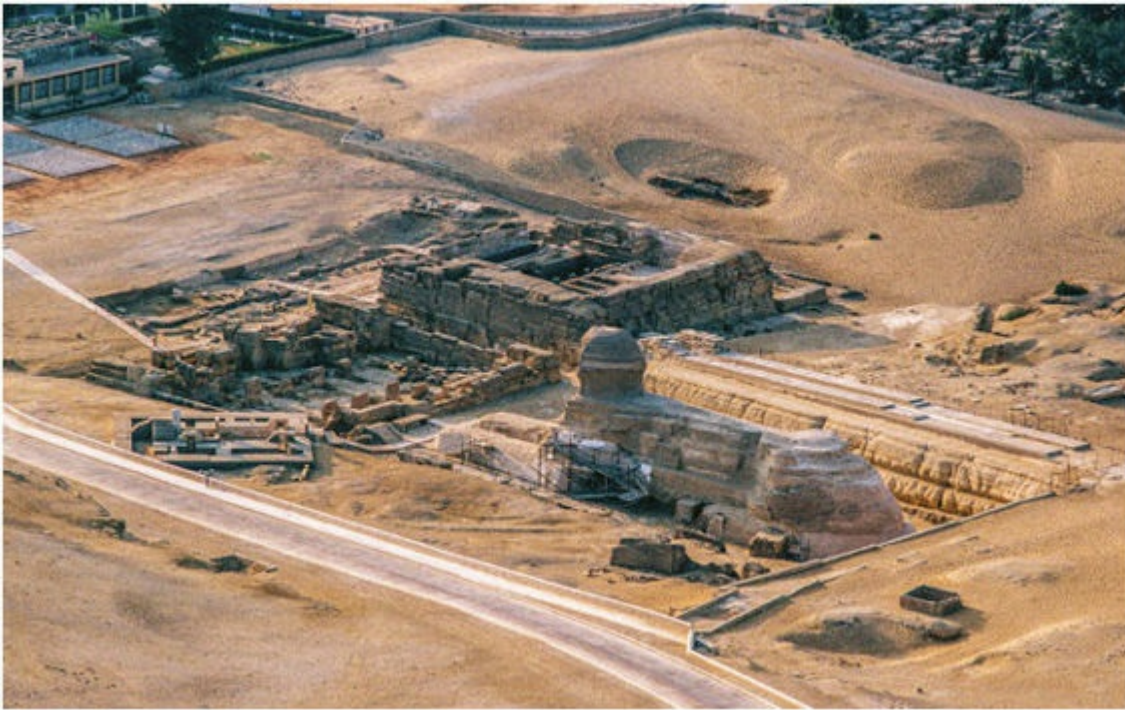
36. The granite elements of the “Valley Temple” were added in Dynastic times to the ancient, preexisting limestone structure.
